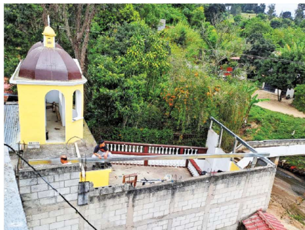
Roof being placed over the new rooms at Los Vados.
